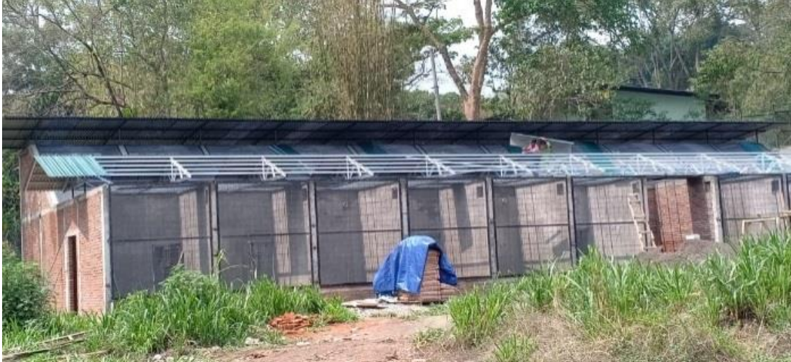
Complex 4, close to the finishing touch
