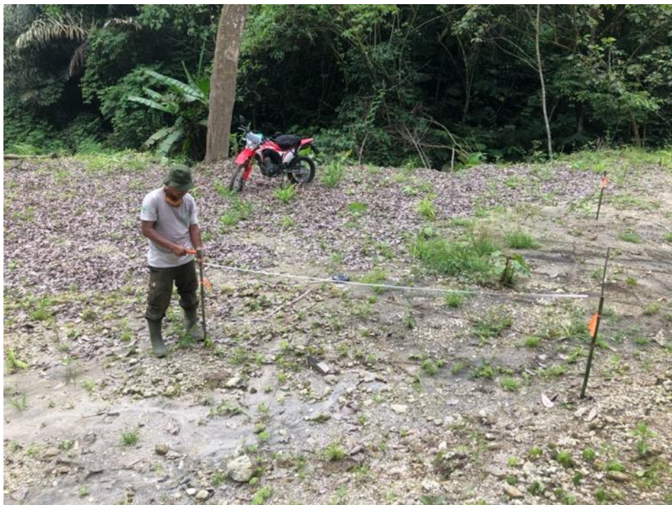
Figures 9 and 10. Ian Singleton and Asril on site, staking out the locations of the corners of the new aviary facility.
