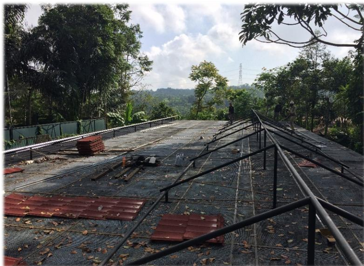
Mesh fitted and roof structure in place
