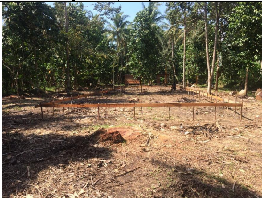
Picture 1: Land prepared, temporary access road created, and perimeter of the clinic building is established - January 2020
