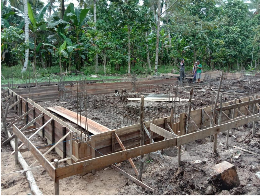
Picture 2: Preparations to pour the cement foundation
