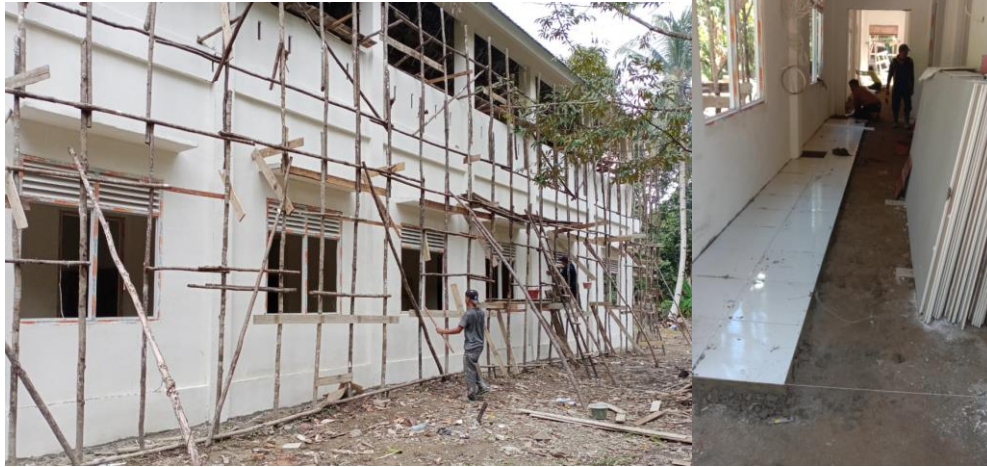
Picture 6: Installation of window frames, drainage system, roof tiles, indoor ceilings, initial paint, and ground floor tiles
