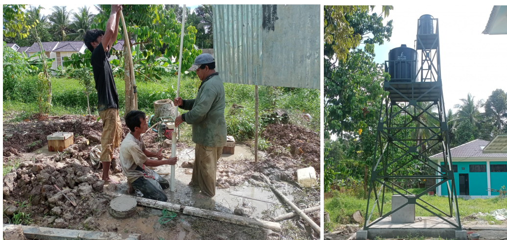
Figure 3: Installation of deep tube-well (left), and overhead water tanks for the rescue center (right).
