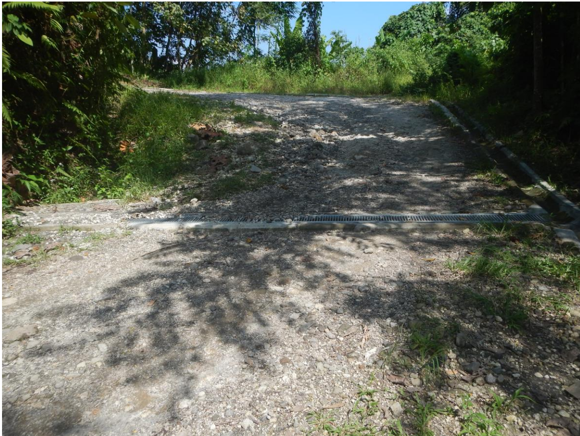
Current road condition without the final layer of paving blocks
