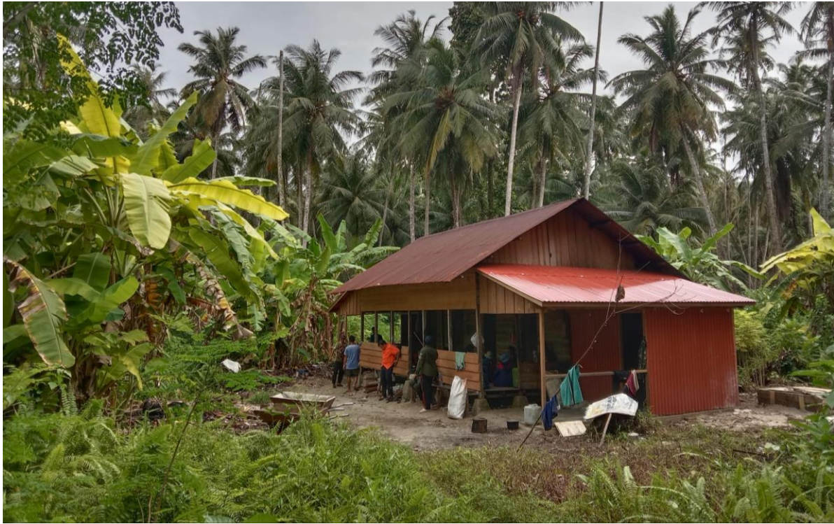
Figure 8. Ranger camp renovation, Linggam Island.
